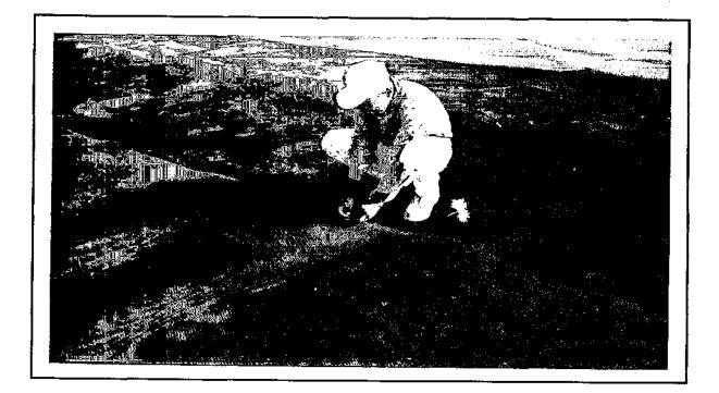
Figure 6.11 - Photograph of Geonet Joining by Using Plastic Fasteners
