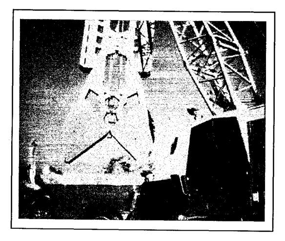
Figure 7.11. Clamshell for Excavating Slurry Trench.
