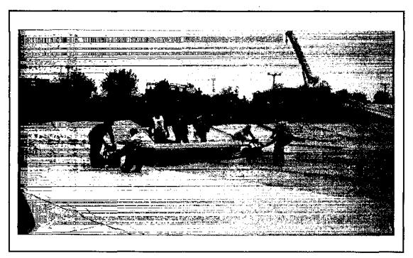
Figure 4.6(b) - Field Deployment of a GCL on an Underlying Geosynthetic
