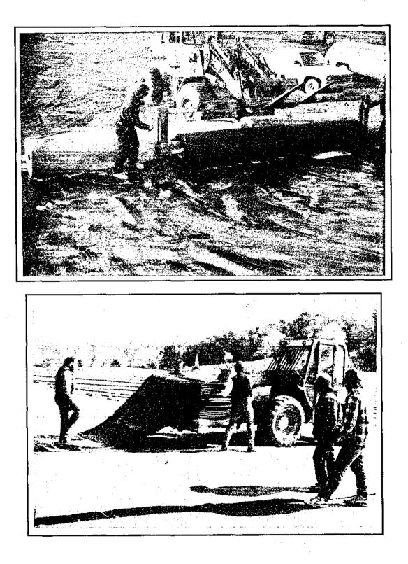
Figure 3.16 - Photographs Showing the Unrolling (Upper) and Unfolding (Lower) of Geomembranes
