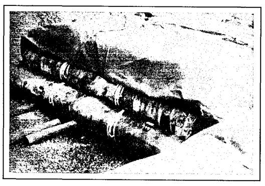
Figure 4.5(b) - Photograph of Temporary Storage of GCLs at Project Site
