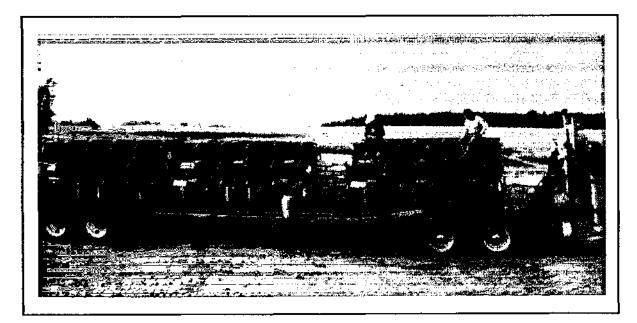
Figure 4.4(b) - GCL Rolls on a Flat-Bed Trailer
