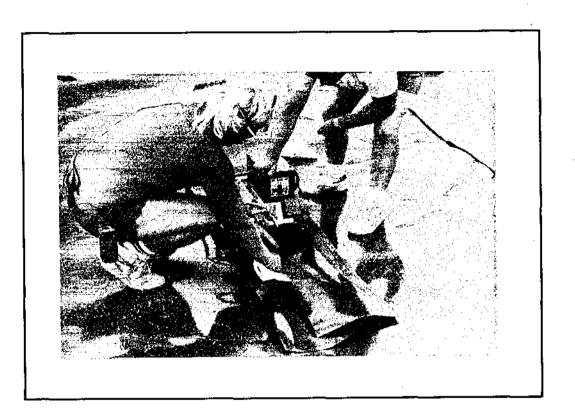
Figure 3.20 - Fabrication of a Geomembrane Test Strip
