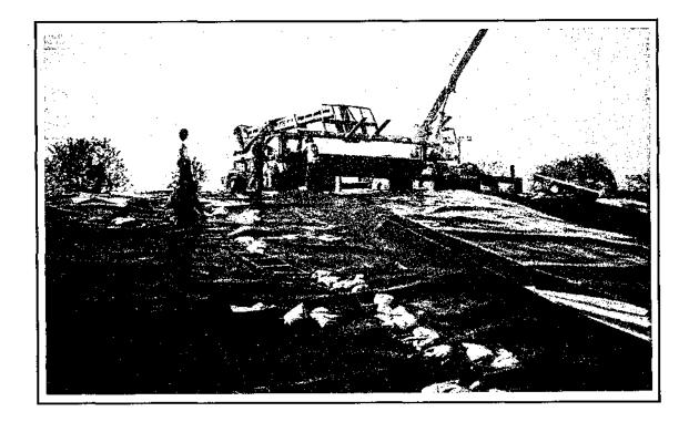
Figure 3.17 - HDPE Geomembrane Showing Sun Induced Wrinkles
