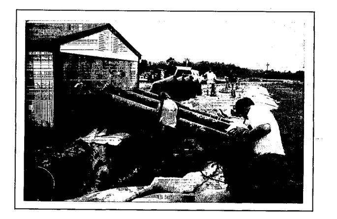
Figure 8.4 - Photograph of HDPE Smooth Wall Pipe Risers Used as Primary and Secondary Removal Systems from Sump Area to Pump and Monitoring Station.
