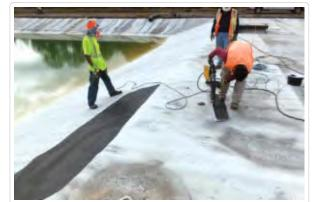
FIGURE 2 Patching a hole in pond liner where a sample was taken for testing in May 2014. The photograph shows trial weld being performed
